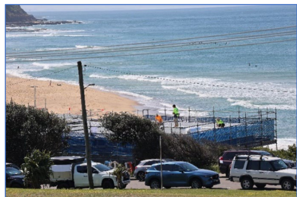
Roof Works at MSLSC – July to November 2025
